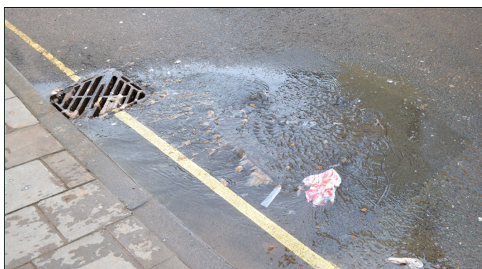
Sewage being discharged in to the drain on Mill Street in Kingsbridge before ending up in the Estuary
