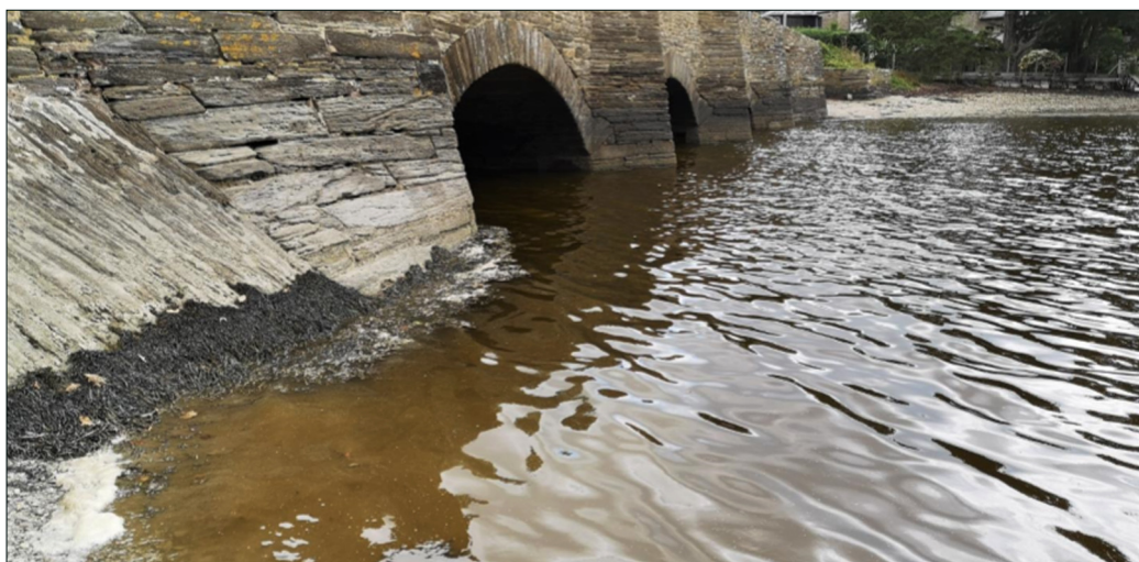
Sewage in Bowcombe Creek by New Bridge September 2019
