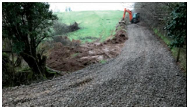
As the photographs above show the track has been constructed without planning permission to a minimum depth of 150mm and immediately adjacent to both trees and hedgerows.
