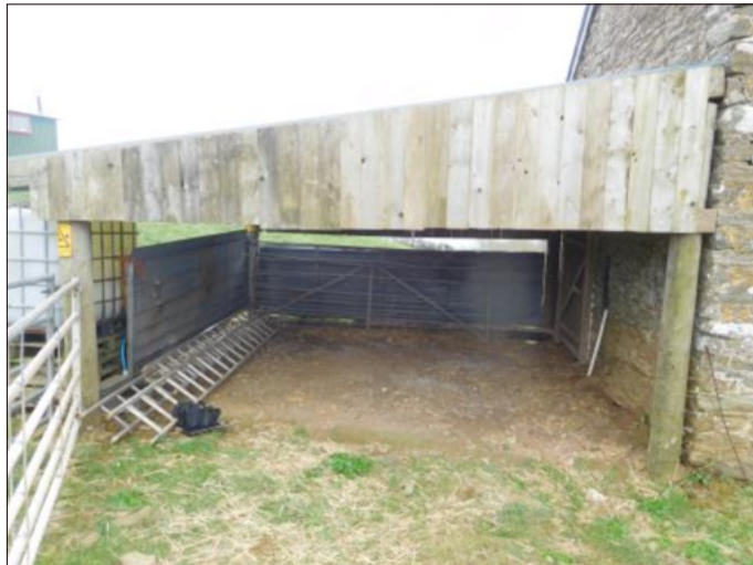
Noticeably no evidence of any agricultural usage
