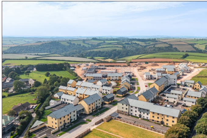
Many will question allowing the erection of architecture from anywhere on green fields in highly prominent locations
