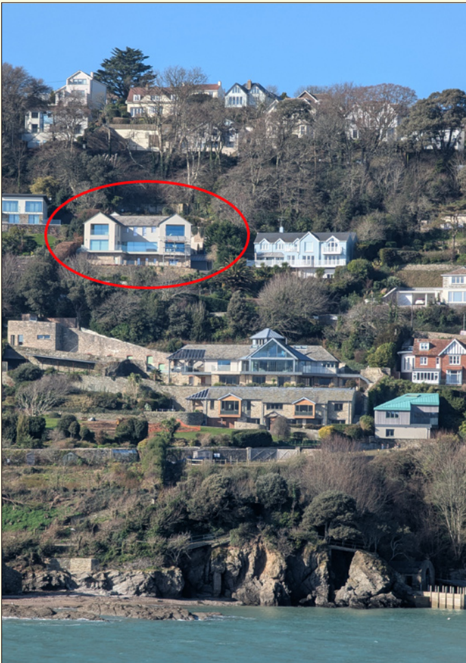
The property: 'much more visible from the estuary'
