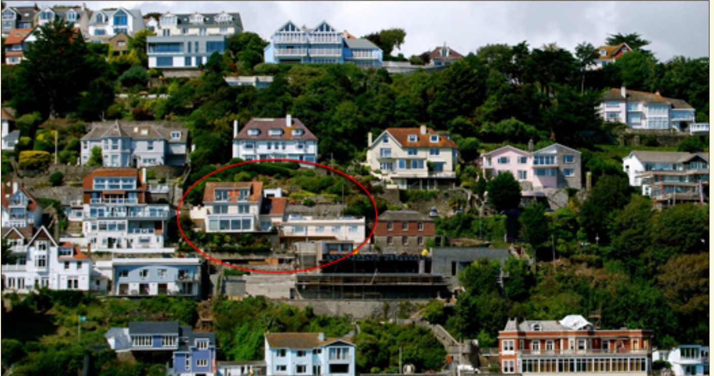
Hillcot as was (above) and today (below). Both its appearance and surroundings have noticeably changed
