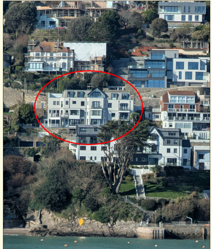
Woodside: further development would make little difference. Inevitably it was approved, and what was previously green was replaced with glazing. •
