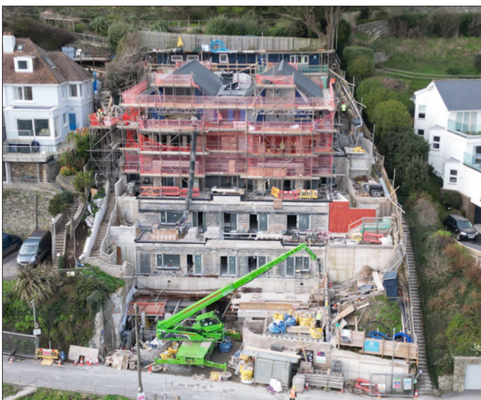
Spion Lodge: more than the one external staircase
