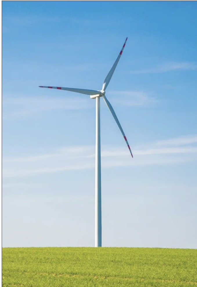
The EWT DW61 1MW turbine, the height to tip of which is 89.5m
