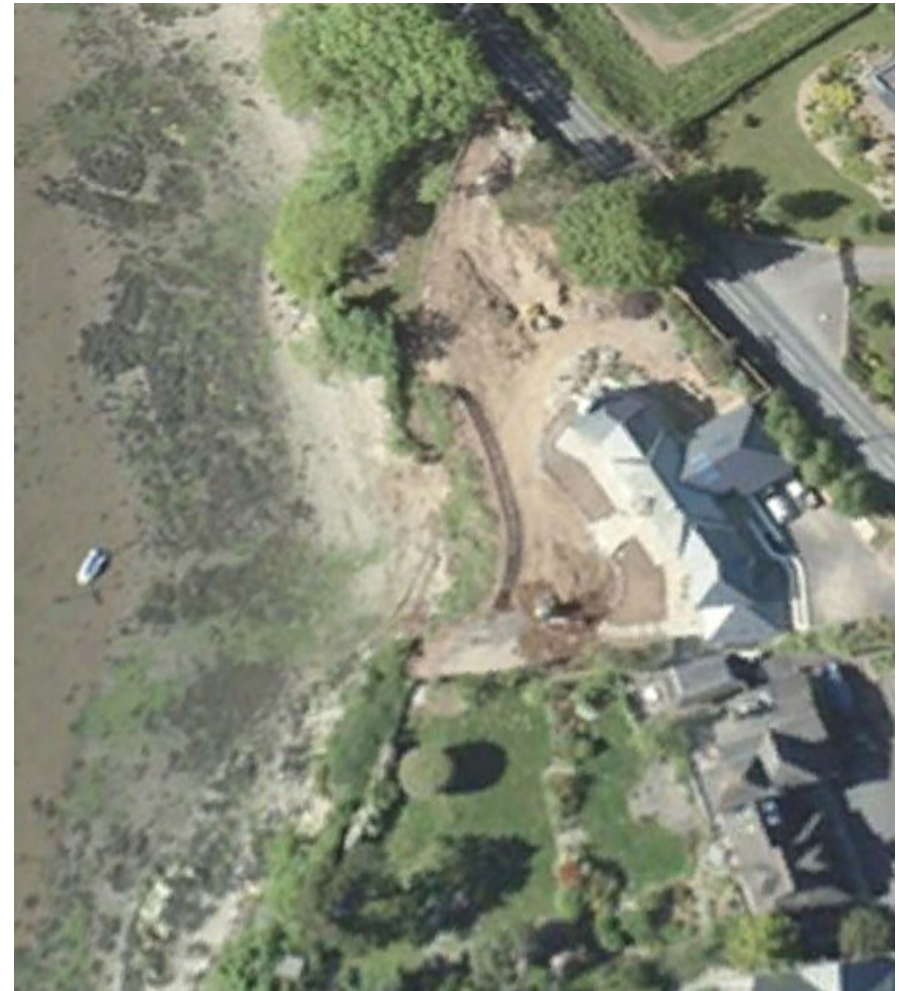
2010, trees along the shoreline removed.
